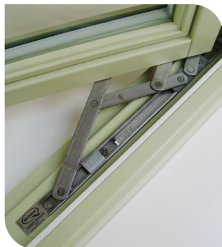
Modern Austenitic stainless steel friction hinges
